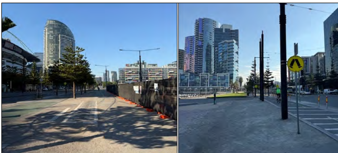
Figure 4 – Views along Harbour Esplanade to the south (left) and north (right) which show the road reserve, bicycle path, old tram tracks and the western footpath directly adjacent to Victoria Harbour (source: CoM site inspections photos taken on 14 March 2025)
